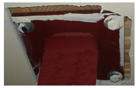
Single Assembly Made from Steel 1/4" (.635cm) Height 10 Feet (3.048 meters) Top Plate: 8" x 8" (20.32cm x 20.32cm) Drilled 4 holes 1" (2.54cm) from Corner Diameter holes 3/4" (1.905cm)
